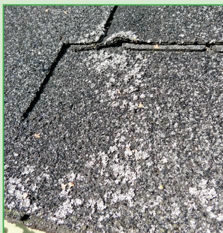
Photo 2: This lichen is growing on an asphalt shingle roof. Lichens generally grow where there's some shade and moist conditions. This side of the roof of this building is partly shaded, an ideal environment for lichens; the other side is in full sun and exhibits no lichen growth.
